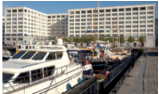
Entrepôt Royal, Anvers – arch. ELD Partnership
